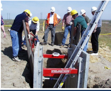
Safety and Rescue Training for high-hazard work activities
